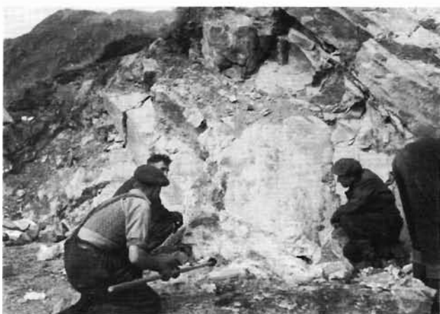
FIGURE 1. View of Sgurr Coire nan Gobhar mica workings, Knoydart. No. 3 Working, Upper Bench, showing highly inclined bands of mica-bearing pegmatite (white) and schist (grey). (BGS Photograph C03796)
