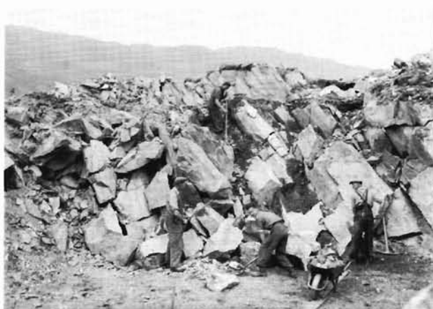
FIGURE 2. View of the Sgurr Coire nan Gobhar mica workings, Knoydart. No. 1 Working, showing workmen excavating mica books from the west end of the Lower Bench. Note the small scale of the workings. (BGS Photograph C03807)
